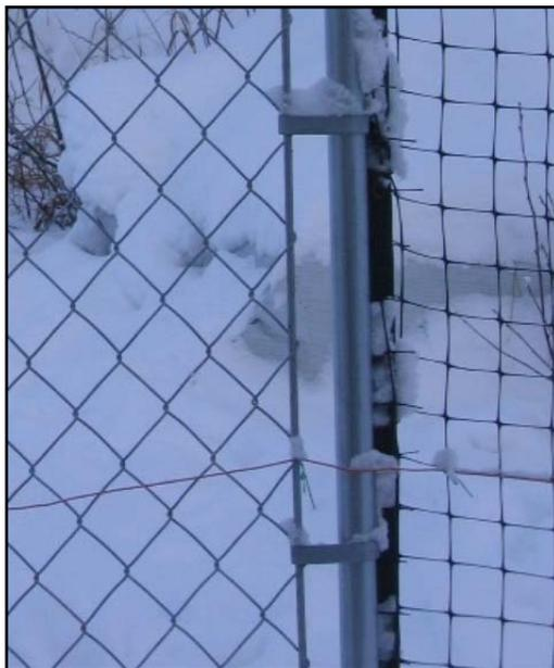
Boundary wire attached to gate and fence
