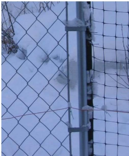
Boundary wire attached to gate and fence
